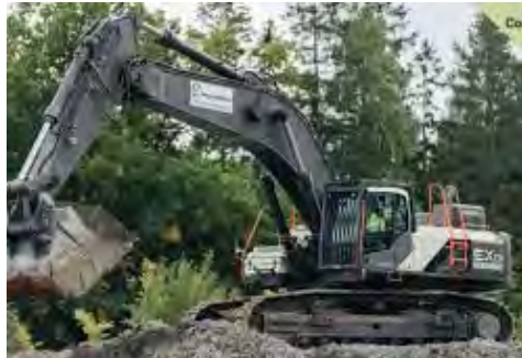
2018: The EX1 - a cable connected excavator
