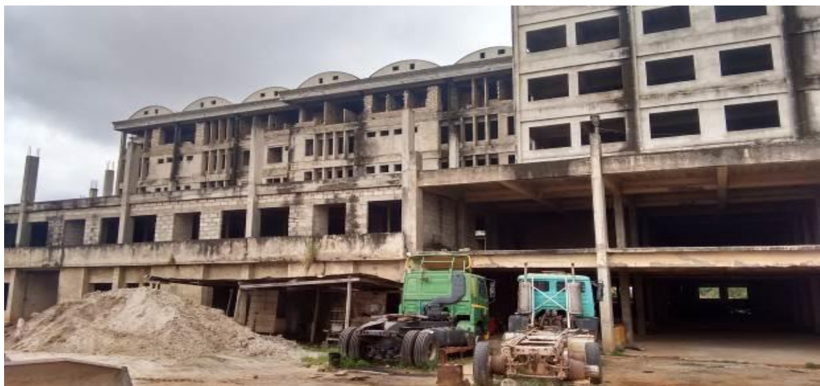
Figure 5 - UNCOMPLETED MATERNITY AND CHILDREN'S BLOCK
