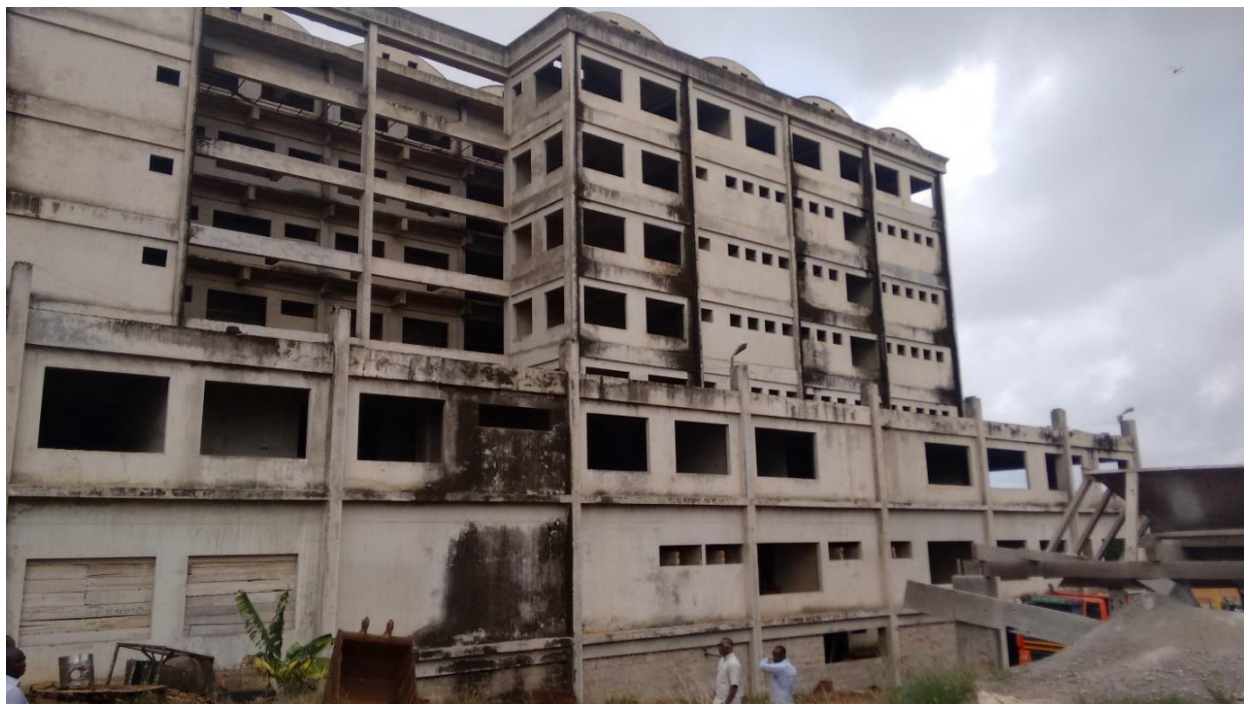
Figure 6 - UNCOMPLETED MATERNITY AND CHILDREN'S BLOCK
