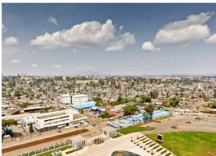
Figure 5: Housing Development Program in Addis Ababa, Ethiopia (Source: iUrban (April 2014): Innovative city strategies for delivering sustainable competitiveness)
