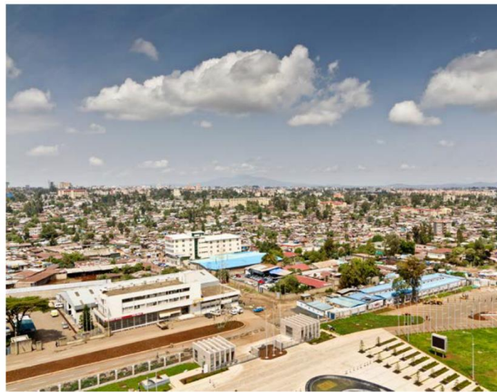
Figure 5: Housing Development Program in Addis Ababa, Ethiopia
